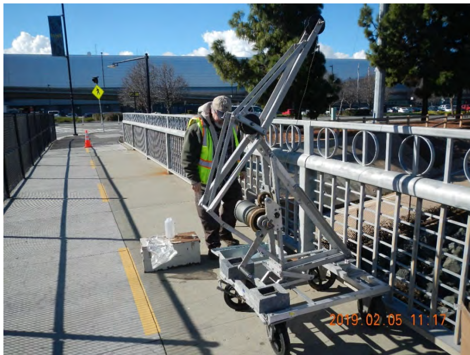
Figure 2-2 D-95 crane set-up adjacent to USGS monitoring gage above Highway 101.
