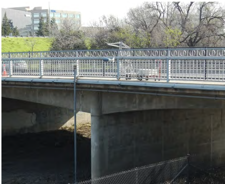
Figure 2-3 View of USGS gage Guadalupe River above Hwy 101 on north side of Airport Parkway bridge and D-95 sampler, looking upstream.
