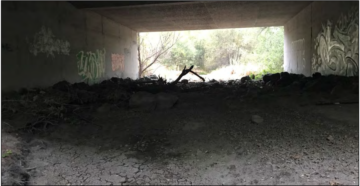
Photo 3. Dry section of Guadalupe River at Foxworthy.
