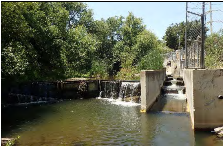
Overview of Guadalupe Creek sampling site.
